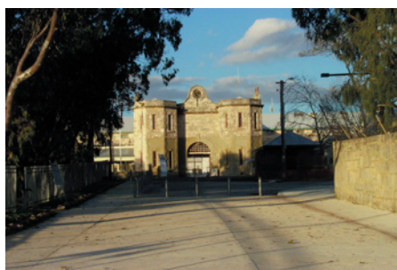
View of Fairbairn Street Ramp looking towards Gatehouse
