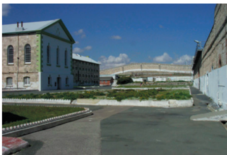
View of the Forecourt and Main Cell Block
