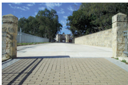
View of the Fairbairn Street Ramp
