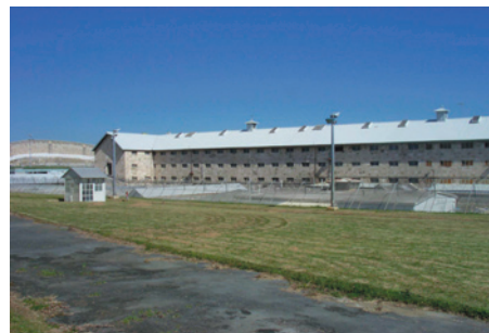
View across the East Terrace to the Main Cell Block
