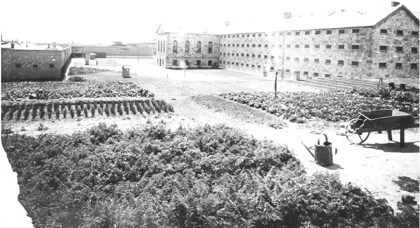
View of Main Cell Block from the South Knoll c1911 Fremantle Prison Collection
