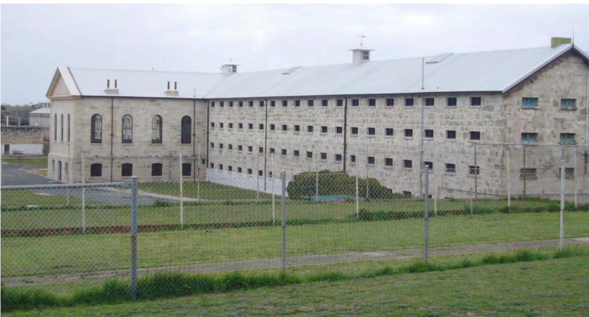
Photographic view of the Main Cell Block from the south knoll, 2007
