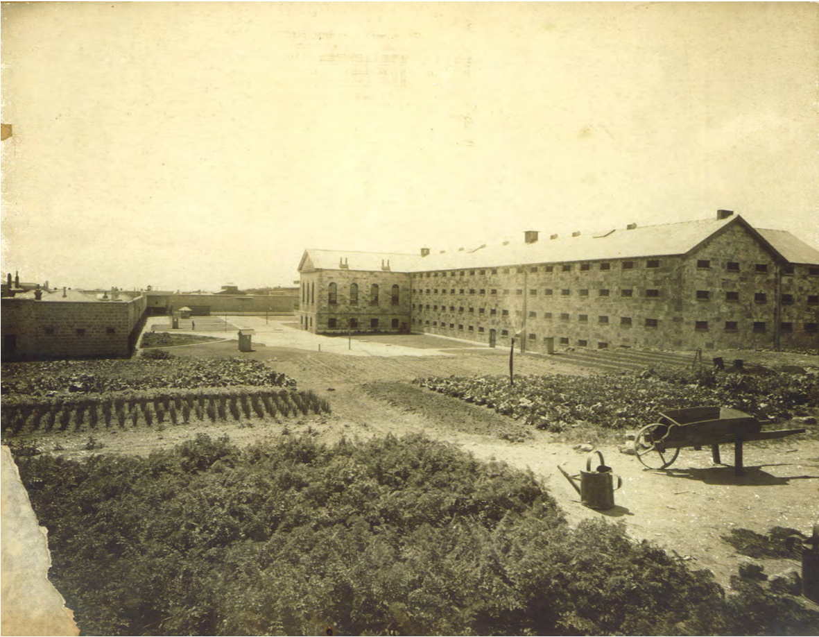
Photographic view of the Main Cell Block from the south knoll, c.1910 (Old Fremantle, J Dowson, 2003)
