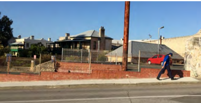
Figure 32. The Terrace, south end, with number 16 at left, number 18 at centre, and the stables to number 18 at right.
