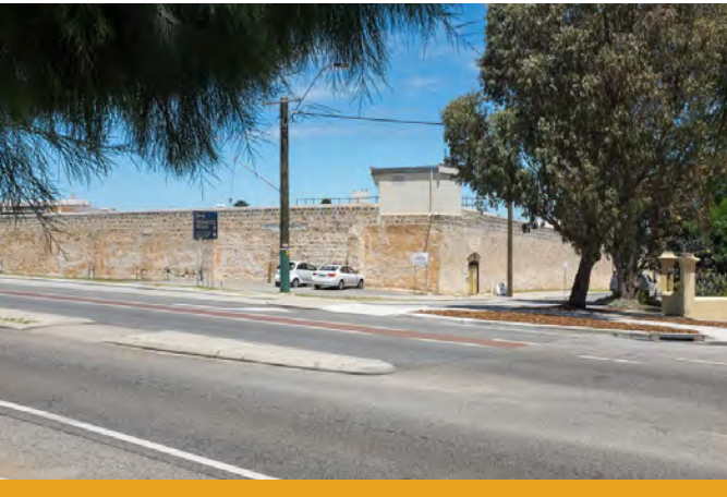
View 3 - This view makes an exceptional contribution to the heritage values of the Prison. New development and plantings should not be introduced to compromise this view.
