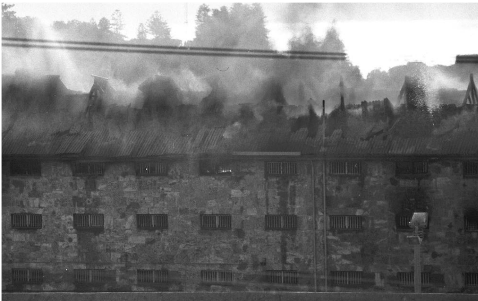
Figure 24. Fire in Main Cell Block during 1988 riot (Source: Reproduced in West Australian, 13 February 2018).
