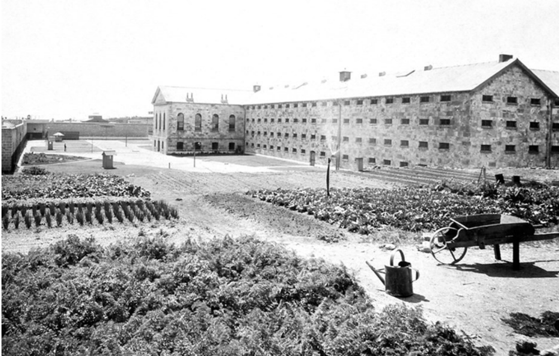
Figure 19. Cultivated gardens at south end of site, part of the reforms during the early 1900s, c1910 (Source: Fremantle Prison Collection).
