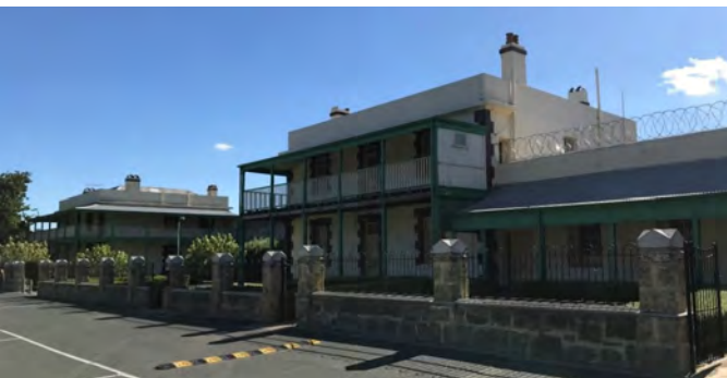
Figure 29. The Terrace, north of the Gatehouse, with number 8 at left and numbers 10 and 12 at right.
