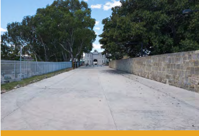
View 23 - Views east to the Gatehouse from the Fairbairn Street Ramp make an exceptional contribution to the heritage values of the place. The views have been compromised to a degree by trees along the Ramp. New development or plantings that may impede these views should be avoided. See 'Overarching Policy – Setting', 'Structures and Spaces Conservation Principles and Actions – The Terrace' and 'Structures and Spaces Conservation Principles and Actions – Fairbairn Street Ramp' for guidance on the management of these views.
