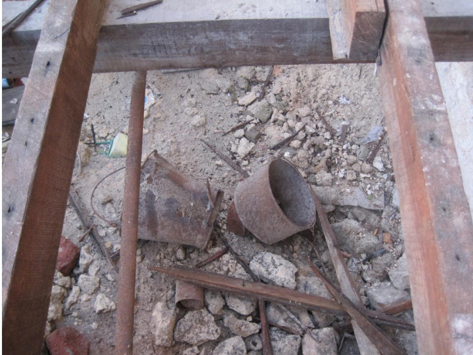
Figure 8 – P877 Warders' Cottages – rear verandah showing example of material under floorboards, including galvanised bucket and pot
