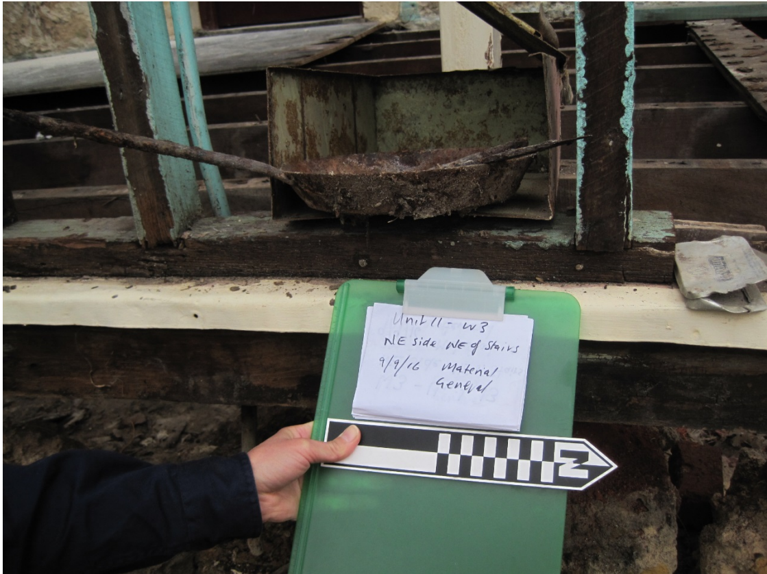
Figure 60 - W3 Unit 11 NE side NE of stairs material general
