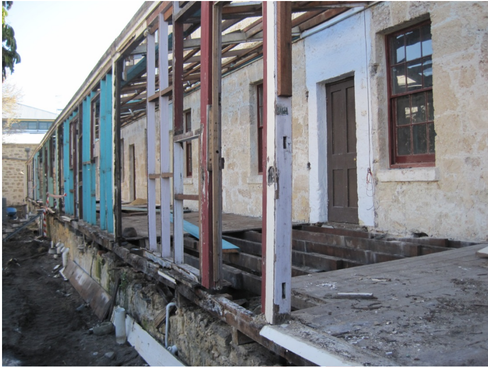
Figure 2 - P877 Warders' Cottages – rear verandahs W3 showing limestone and brick wall
