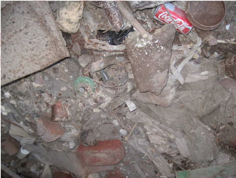
Figure 9 – P877 Warders' Cottages – rear verandah showing example of material under floorboards, including pot lid, fragmentary refuse, and coke can
