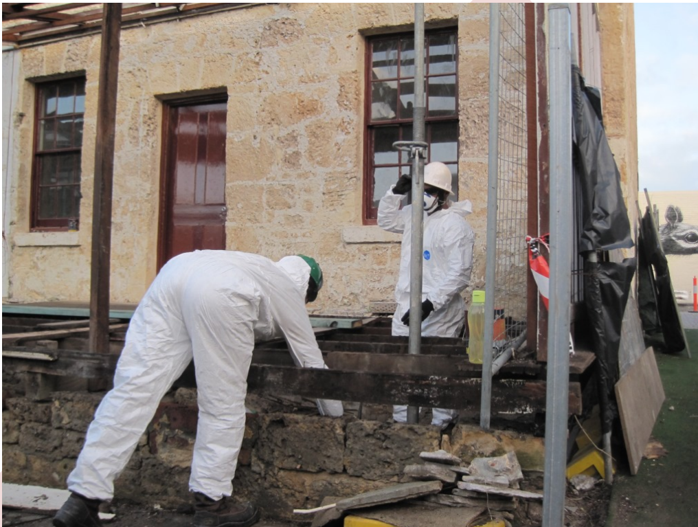
Figure 13 – W3 Unit 17 Showing contractors recovering material
