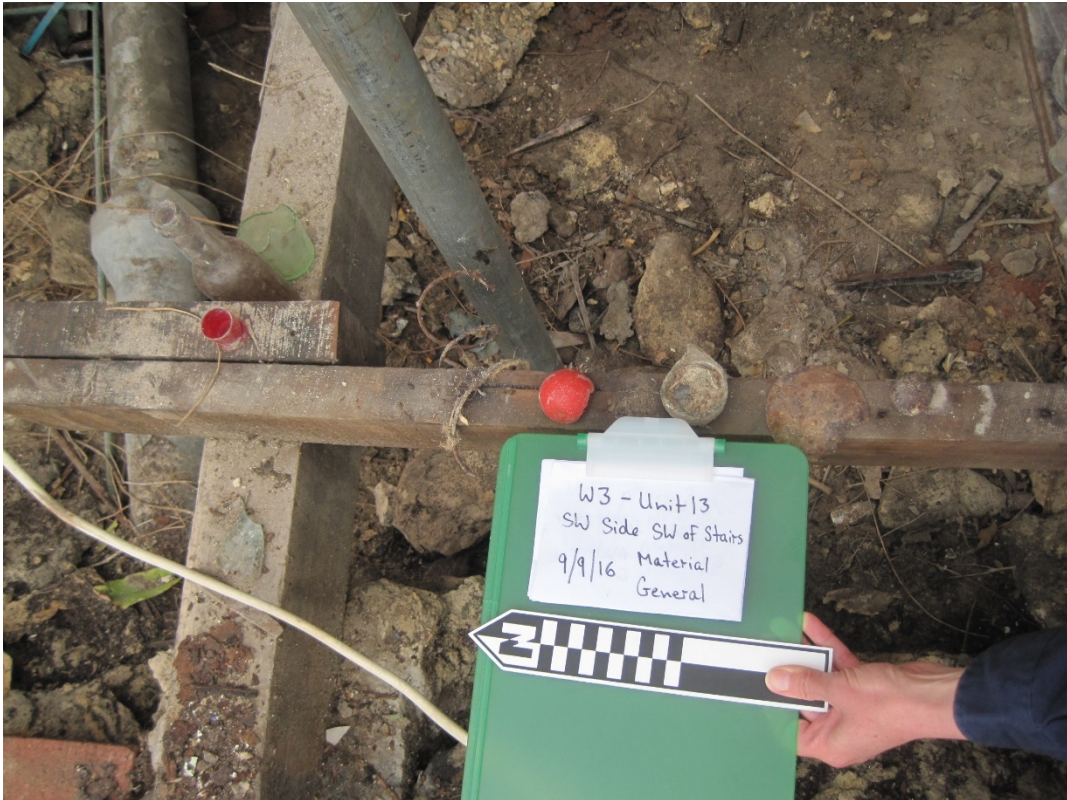
Figure 94 - W3 Unit 13 SW side SW of stairs material general
