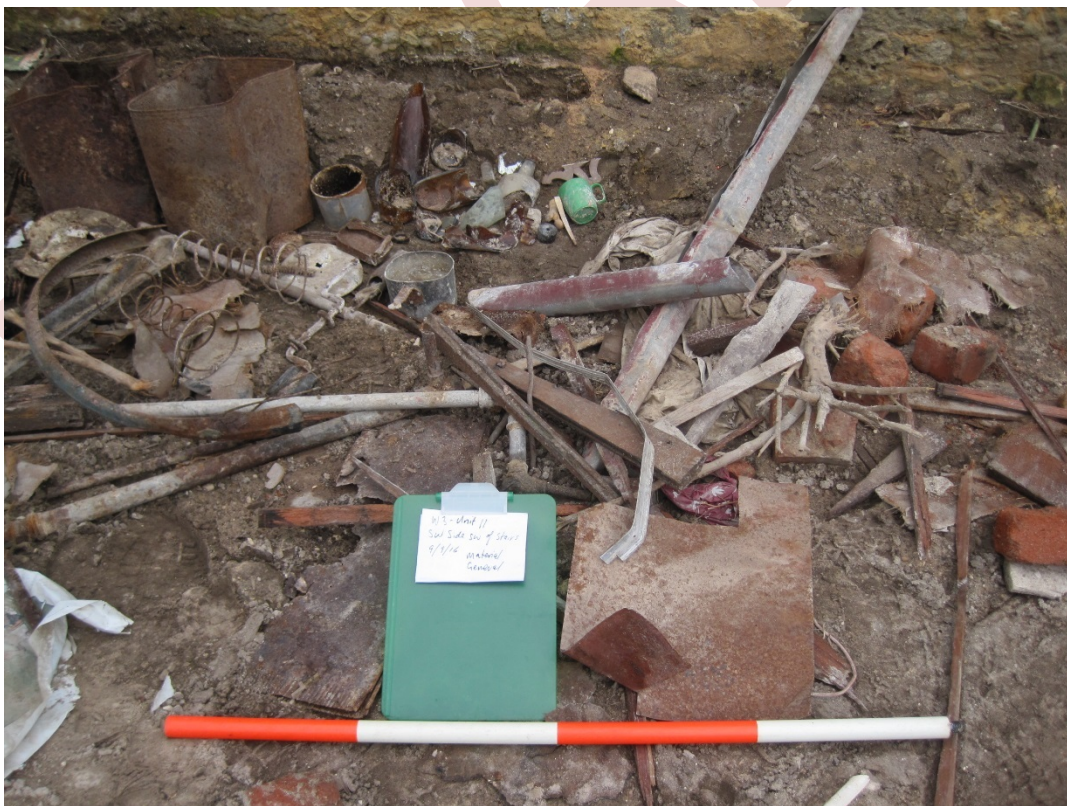
Figure 73 - W3 Unit 11 SW side SW of stairs material general
