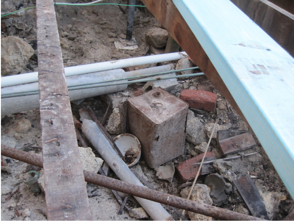
Figure 6 – P877 Warders' Cottages – rear verandah showing example of material under floorboards, including enamel bowl and kerosene can
