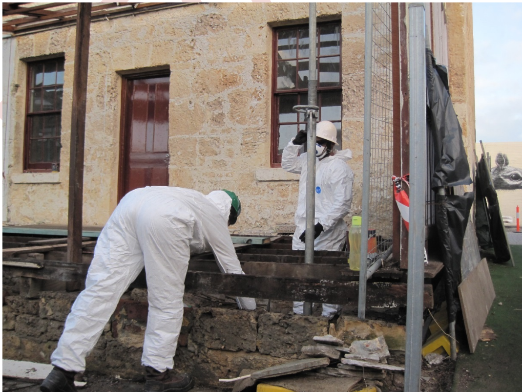
Figure 107 - W3 Unit 17 Contractors commencing refuse removal
