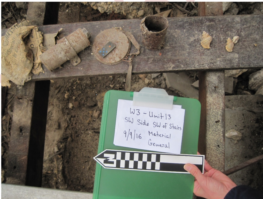
Figure 93 - W3 Unit 13 SW side SW of stairs material general
