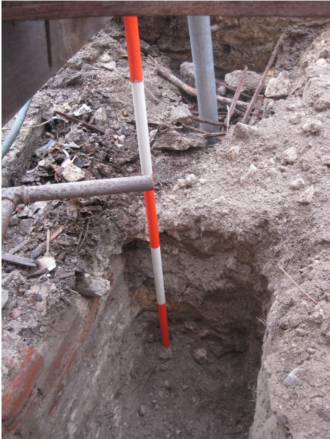
Figure 29 – Firewall trench 5, final excavation depth
