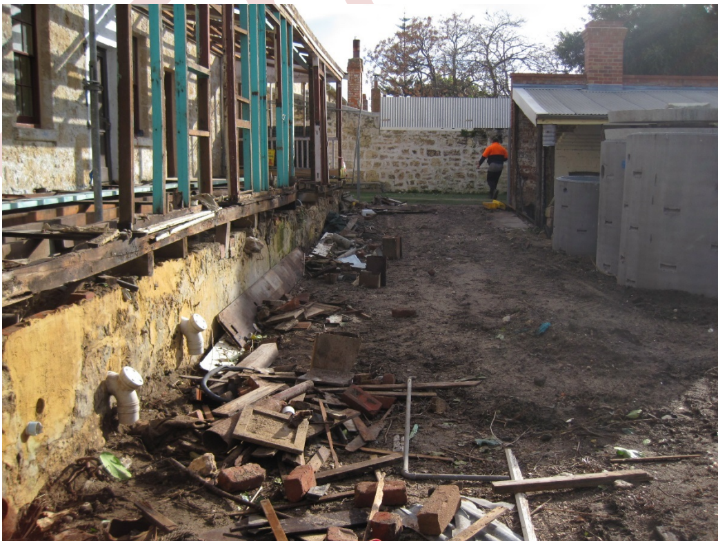
Figure 31 - W3 View to NE towards Fremantle Market Laneway
