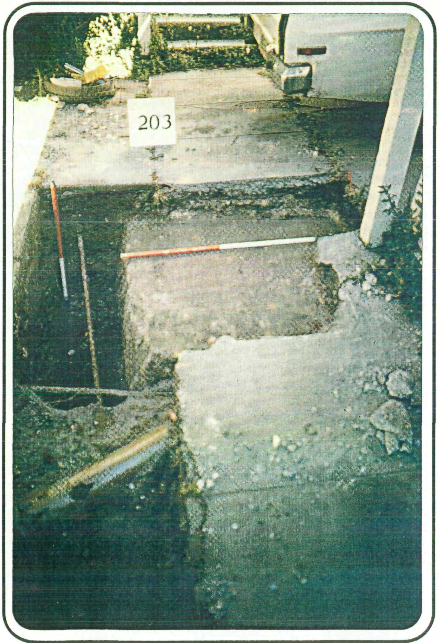
TEST PIT 200, FOUNDATIONS 203, VIEW NW
