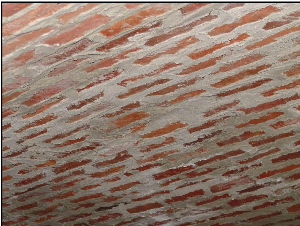
Plate 2: Arched brick ceiling in No. 14 cellar
