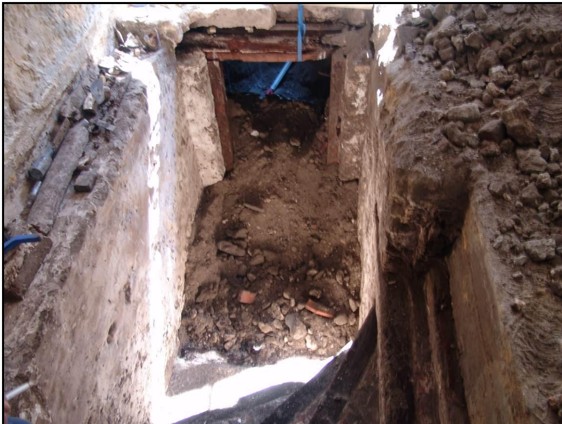
Plate 4: View west down stairwell to cellar door
