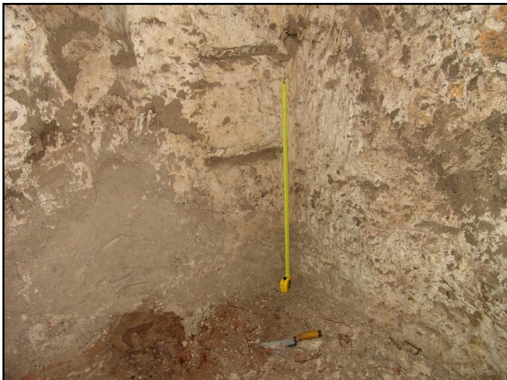
Plate 5: Notches for shelving cut into cellar wall
