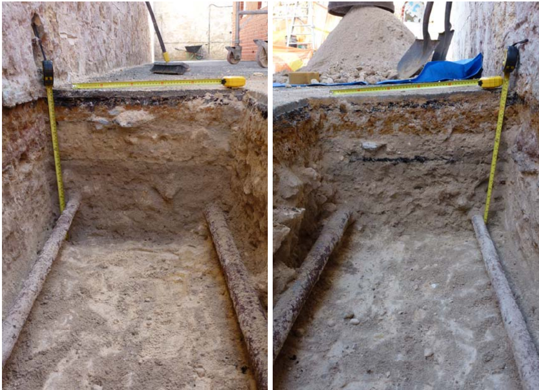
Plate 8: View of SW corner of trench, showing base of red/pink render on S wall (red line) and base of limestone deposit 004 on E facing section (white line).
