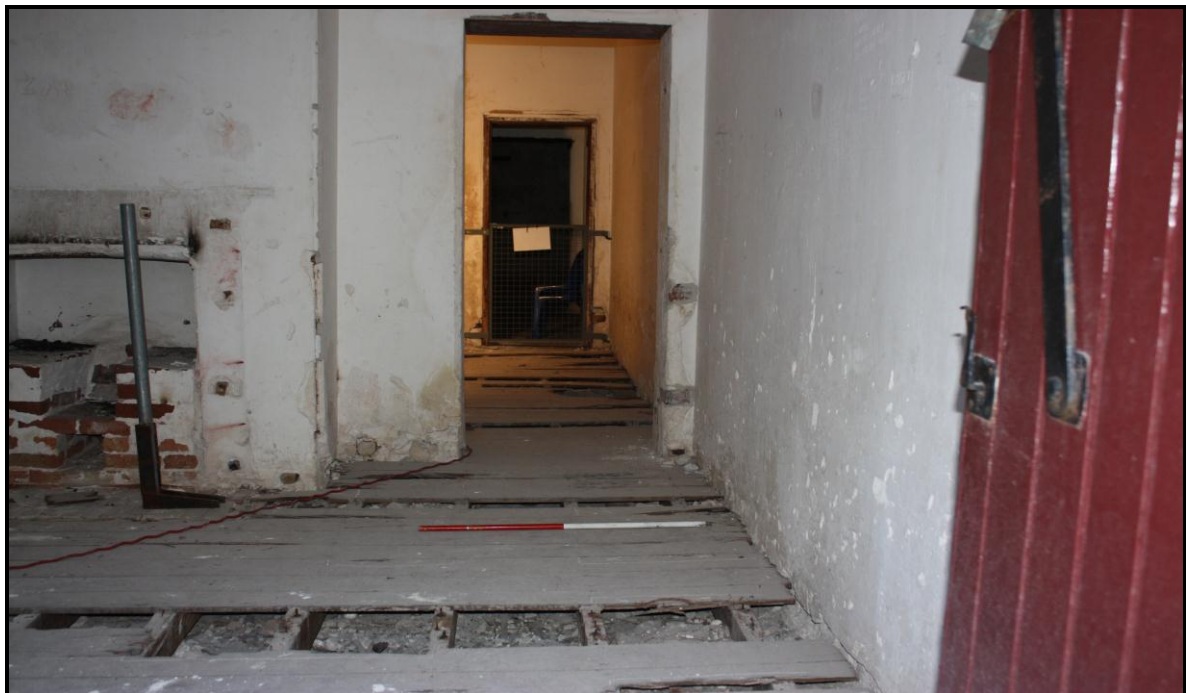
Plate 1. View east through the steward's office to the clerk's office (Scale = 1m)
