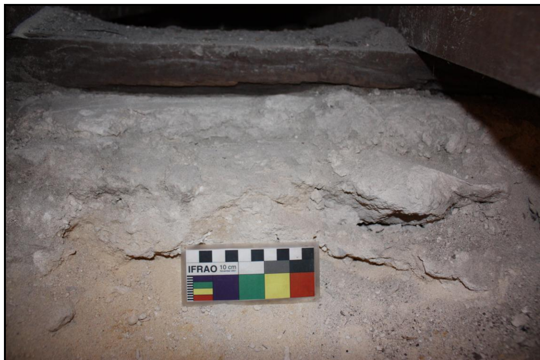
Plate 3. Slot 1, profile showing jarrah beam and lime mortar pad, view west (Scale = 10cm)
