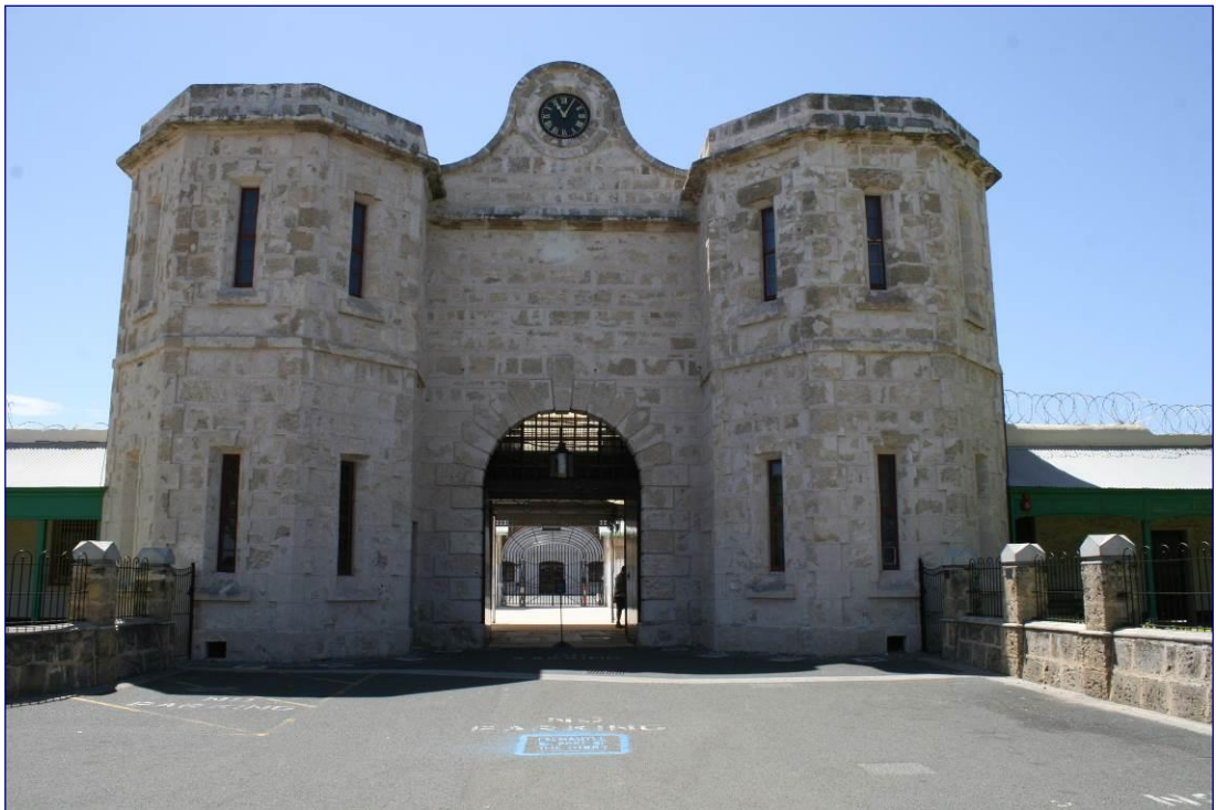
Figure 1.1 The main gate to Fremantle Prison, facing east.
