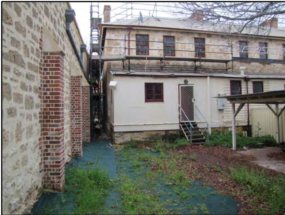
Plate 9: View NW of rear yard of cottage, block W3, house 7
