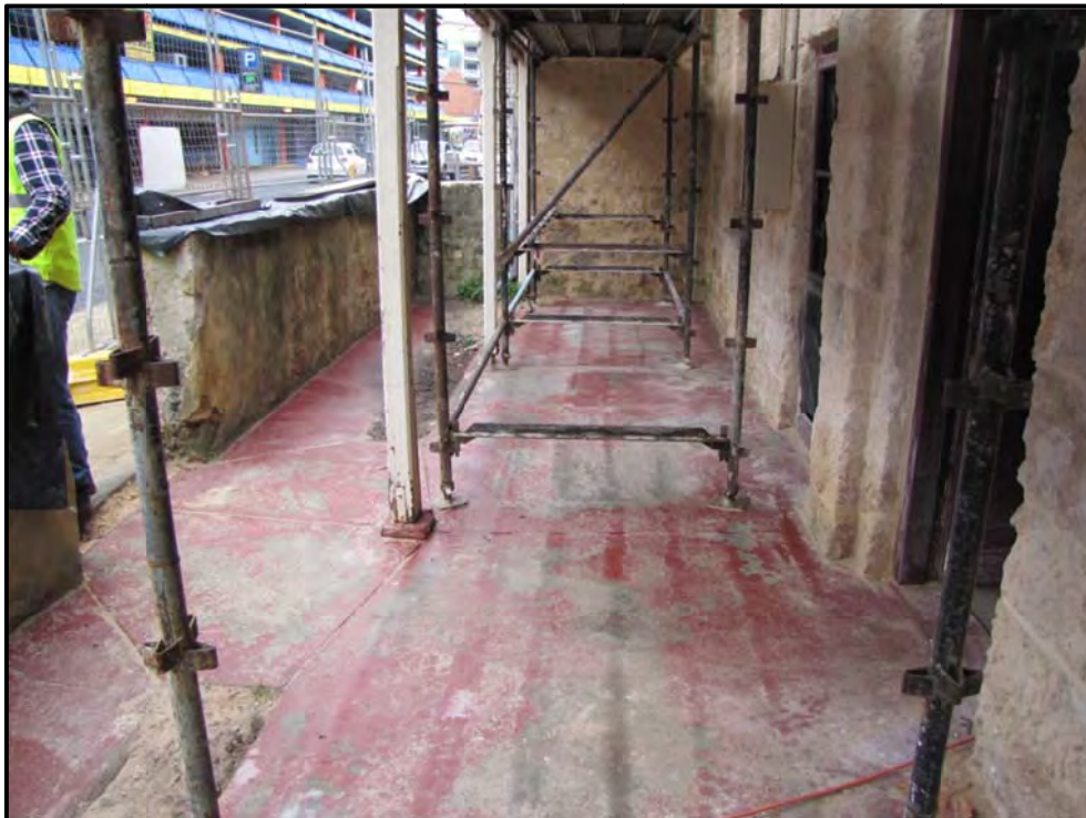
Plate 1: View NE of concrete front verandah, block W2, house 39/41
