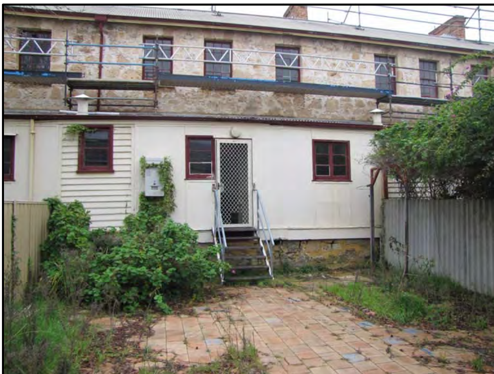
Plate 8: View NW of rear yard and façade of cottage, block W3, house 11
