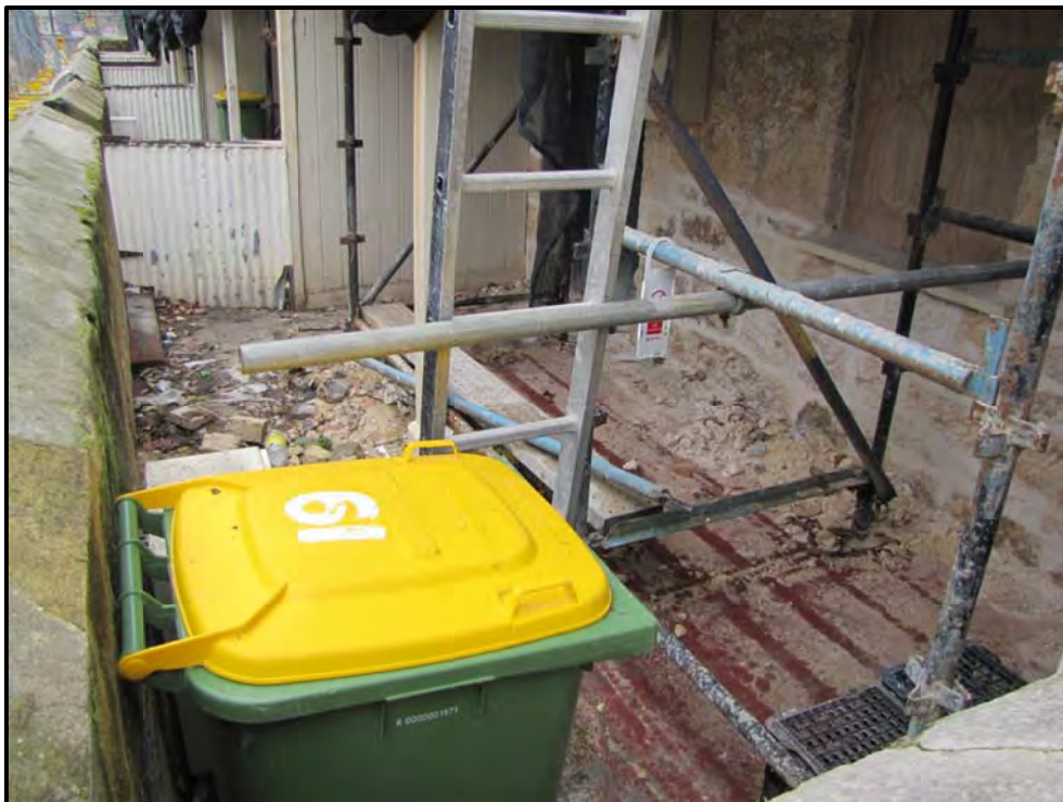
Plate 10: View E/NE of concrete front verandah, block W1, house 19
