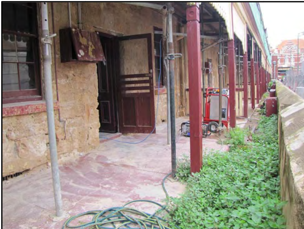
Plate 11: View SW along concrete front verandahs of block W3
