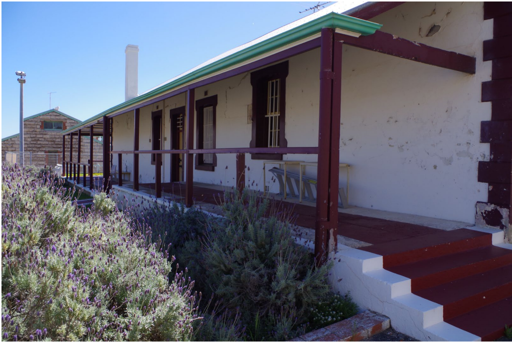
Plate 1: - Southeast section of verandah, F. Jose, 2020
